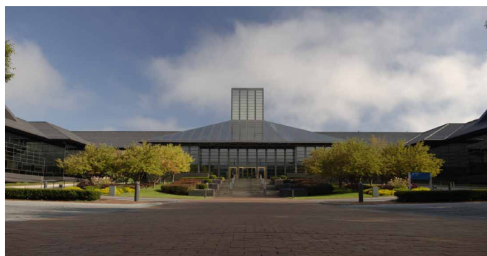
Corning Inc.'s headquarters building in Corning, NY.
